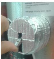
**STEP 3**Remove adhesive tape liner and fit the duct-tape to the tube.
