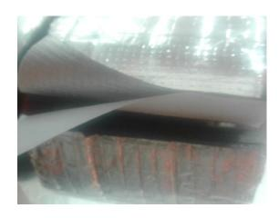
**STEP 6**Secure the insulation cap by applying the duct-tape supplied with the kit.
