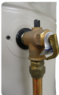
TPR position - top of cylinder
